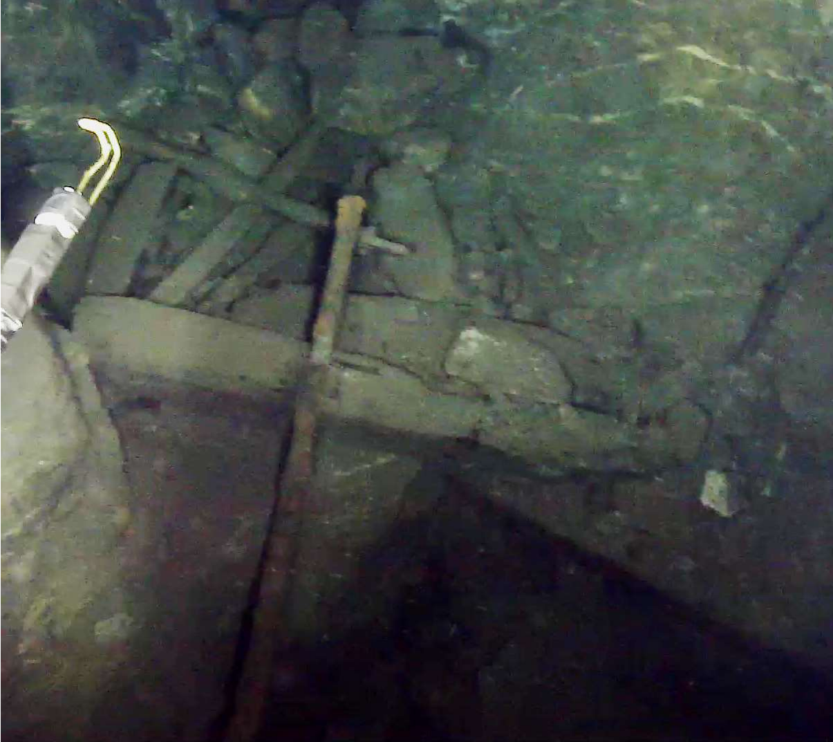
Plate 24: Displaced timberwork on the floor of the entrance to the NW4 eastern trial near the present North Winze base. This is overlain by a modern scaffold pole in the shaft. To the bottom right in the gloom is the horizontal timber that is either also displaced or was a 1790s support for a platform across the shaft at the horizon of the floors of the short NW4-5 'trials levels' leading east and west.
