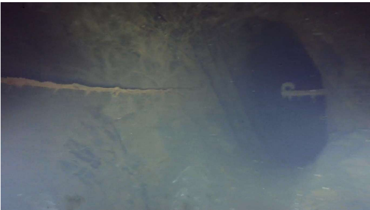
Plate 20: The metal chain across the large 'pipe working' that runs WNW from the PW1 upper chamber in the 'main pipe working'. The camera is looking into the 'cross cut' running NNW. The chain provided a 'hand-rail' for a bridge near the 'pipe working' roof, with a hook on the opposite side for a second chain. Presumably there was once a timber that was used to walk on
