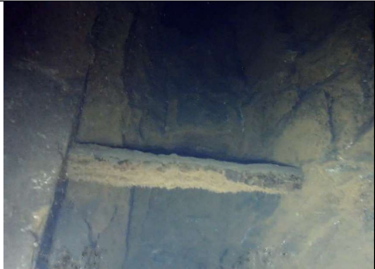
Plate 22: A timber beam, presumably for a working platform, in the tall alcove near the north-eastern corner of the upper 'main pipe working' chamber at PW1
