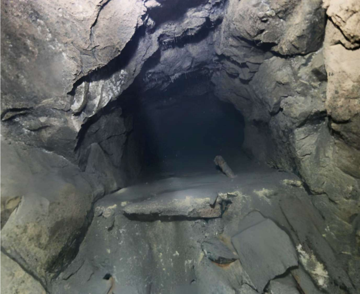
Plate 26: This small, part-backfilled WS1 'level' heads north from the winding shaft at a point only just below c. -5.0m from the shaft top. It has not been entered and while it is heading towards the pumping shaft there is no matching opening at this depth and thus its destination is elsewhere
