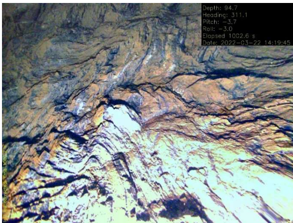
Plate 8: Disharmonic folding in thinly bedded limestones in the wall of the pumping shaft at -94.7m depth
