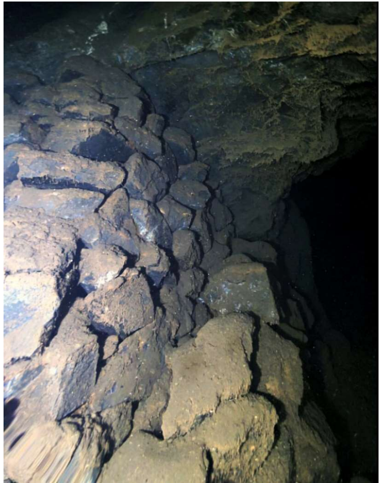
Plate 17: One of the packs of deads at PW11B, with a bedrock pillar behind, and to the right one of the openings that has not yet been explored but probably goes to the PS8 'side pipe workings' at the side of the pumping shaft
