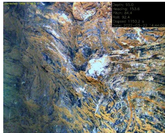
Plate 9: Further disharmonic folding in thinly bedded limestones in the wall of the pumping shaft at -95.0m depth
