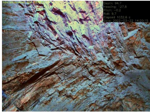
Plate 7: Another fracture in the axial plane of a small-scale syncline in the wall of the pumping shaft at -94.7m depth
