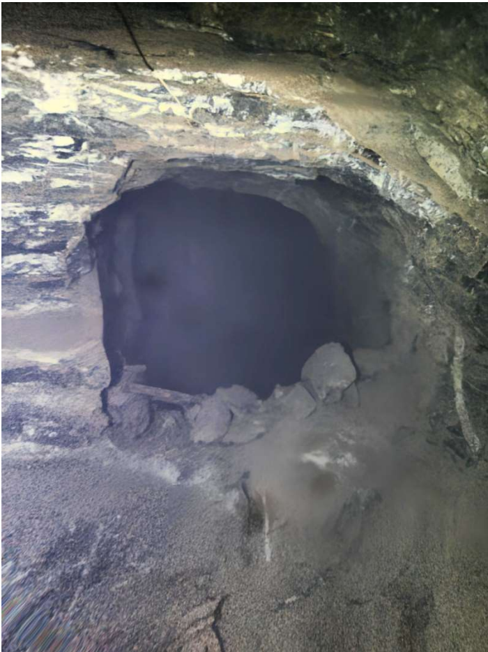
Plate 15: The WS5 opening looked at from the PW6 'main pipe working', with the side walls of the winding shaft just visible behind the rubble-covered ledge between the two features.
