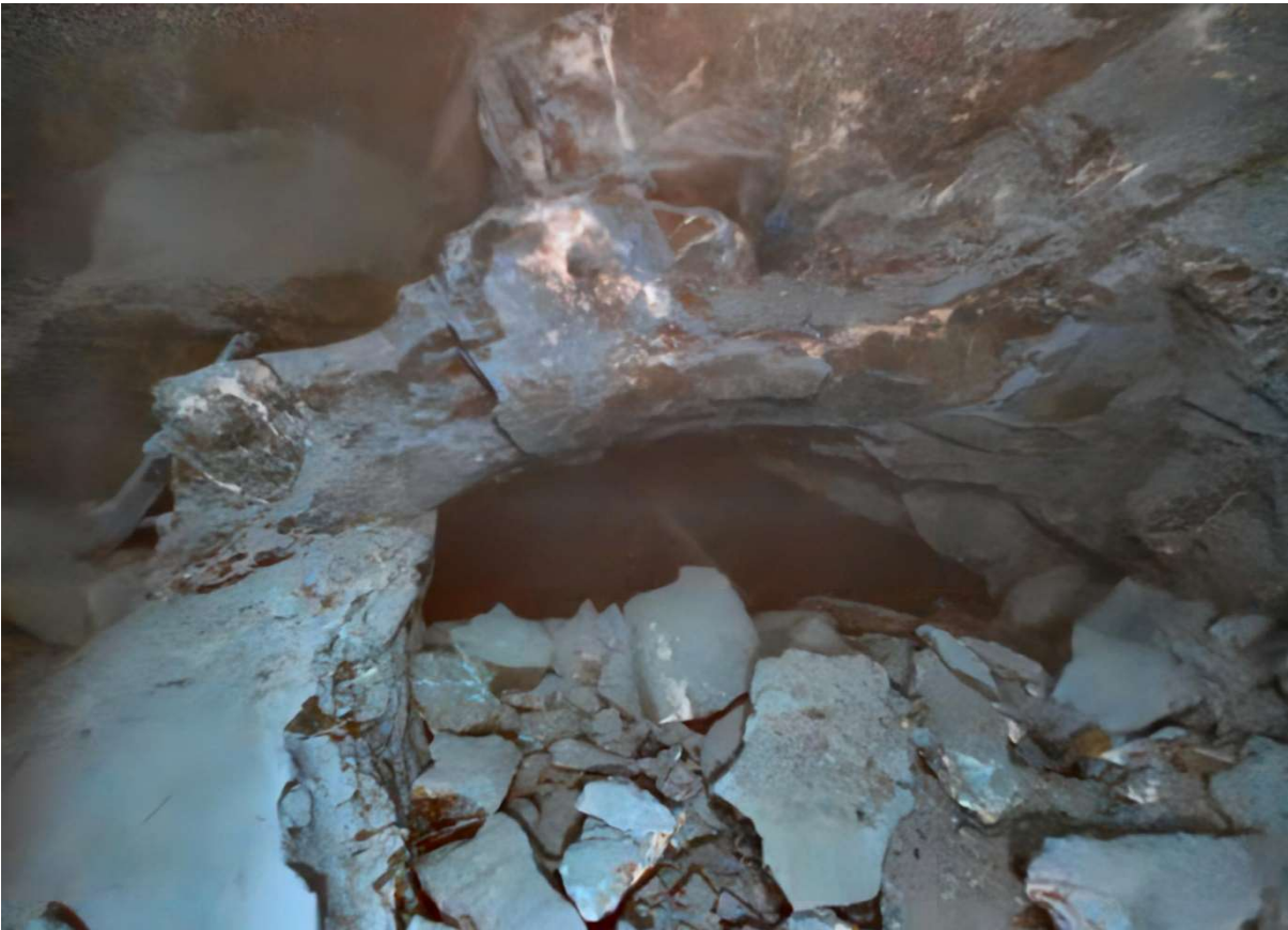
Plate 12: The open part of the PS9 'level' or 'side pipe working' at the south-east end of the pumping shaft. Much of the passage is filled with rubble and, out of shot, there is a complex arrangement of in-situ timbers supporting this backfill at the shaft wall; in total the passage was originally 2.5m high, with a roof at -58m and floor at -61.5m down the shaft. The passage has an unknown destination, but this is possibly the 'main pipe working' or it was a 'cross cut' to the documented 'Deep Level' at -62m. To the left is the large PS8 'side pipe working' lying at the north-east side of the shaft.
