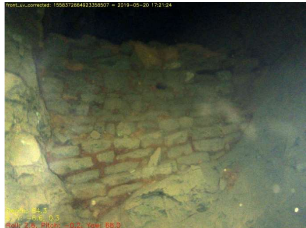
Figure 11. The carefully-built wall across a passage intersected by the pumping shaft at 65m below water level, with what appears to be clay in the interstices, appears to have been built as a dam to hold water back. Possibly the Ape Tor boat level
