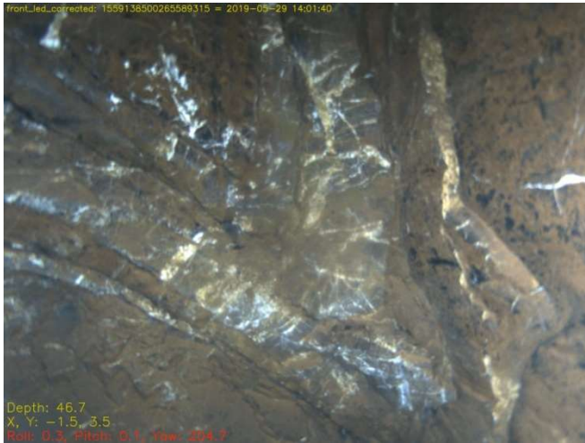
Figure 3 Tight syncline in limestone at 46m depth below water level in the Ecton winding shaft
