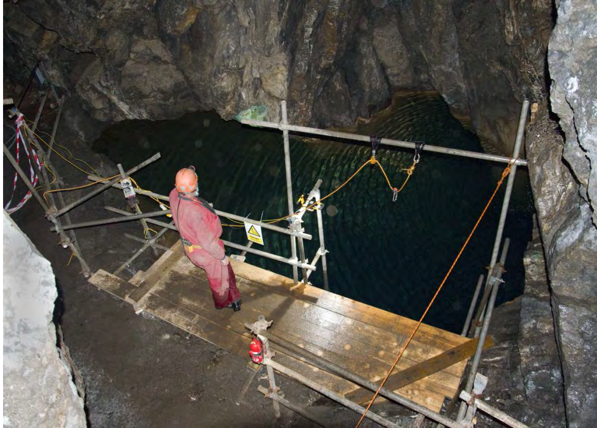
Fig. 7.47: The launch platform at the ‘main pipe working’ ready for use (Photograph: John Barnatt).
