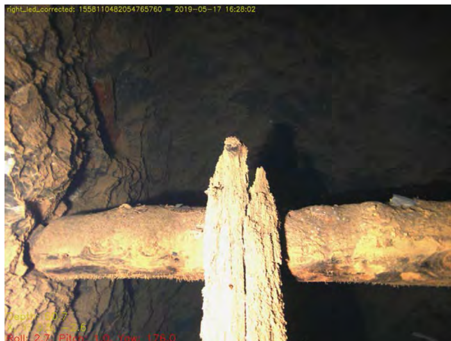
Fig. 7.31: One end of the timber at PS10 at the north-western end of the pumping shaft; the timber resting on it is the once-vertical one at PS11 that lies at the other end of the shaft, which has fallen across the shaft and come to rest on the PS10 timber above. The end of the PS10 timber has been shaped to fit into a small cut ‘ eye ’ in the shaft wall.
