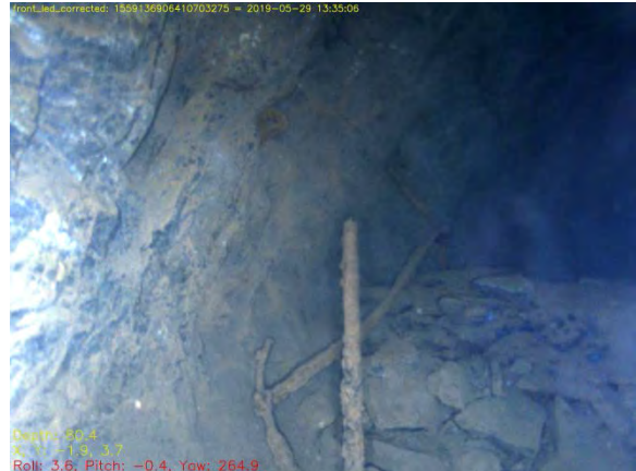
Fig. 7.46: The iron bar with two curved end pieces, behind a metal pipe, at the winding shaft edge in the WS8 cross-cut from the pumping shaft. This may have fallen down the shaft and was perhaps a tie-bar that was once fastened to a large timber structure. There is also an iron ‘eye’ above that is fastened to the wall at the level entrance.
