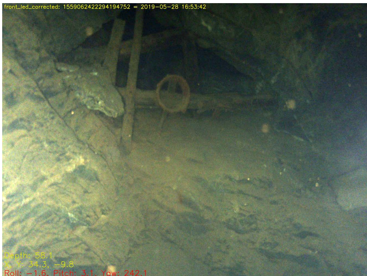
Fig. 7.38: The ‘side pipe working’ at WS6, with collapsed support timbers and a metal drum within its entrance, photographed from within the winding shaft. The timbers are likely to have fallen from higher within the ‘side pipe working’, with the drum placed here at a later date.
