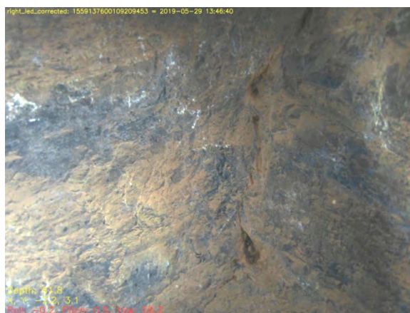
Figure 8.1.25 Oxidised sulphide blobs in fracture plane. Winding shaft -61m.
