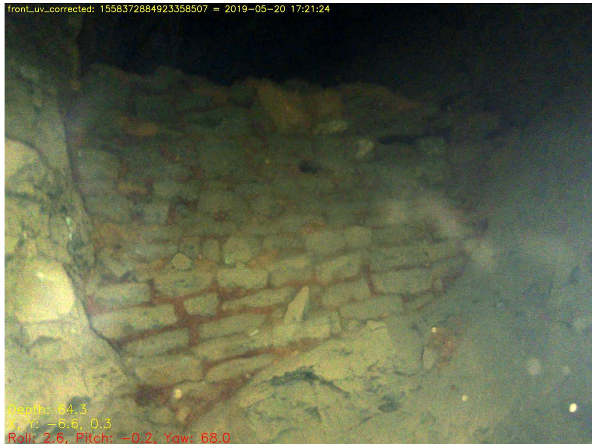
Fig. 7.27: The carefully-built dam across the passage at PS12, with what appears to be clay in the interstices, looks to have been built as a dam to hold water back; the text explores several potential explanations for why this was created.
