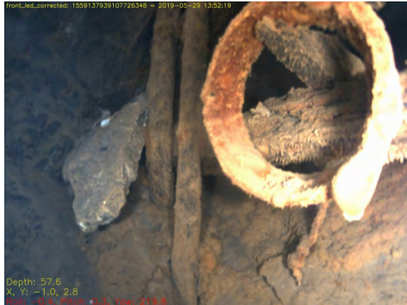
Fig. 7.45: The iron ‘drum’ at the WS6 ‘side pipe workings’, resting on one of the collapsed timbers. Its position may suggest it has been purposefully placed here rather than coming to rest on the timber after falling down the shaft.
