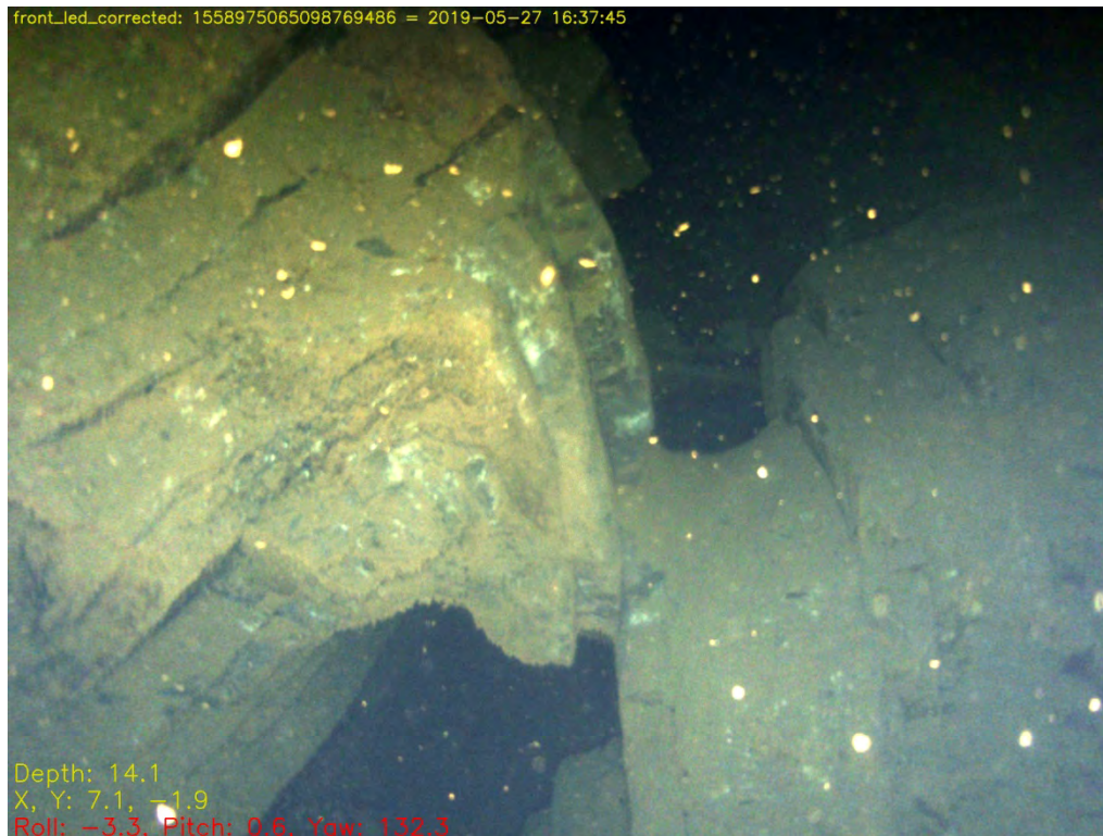
Fig. 7.63: A detail, captured in the gloom, of the complex area of passages at PW3 between the upper and lower passages with many interlinked passages, here with a small rock bridge left by the miners at the top of a fold in the limestone beds.
