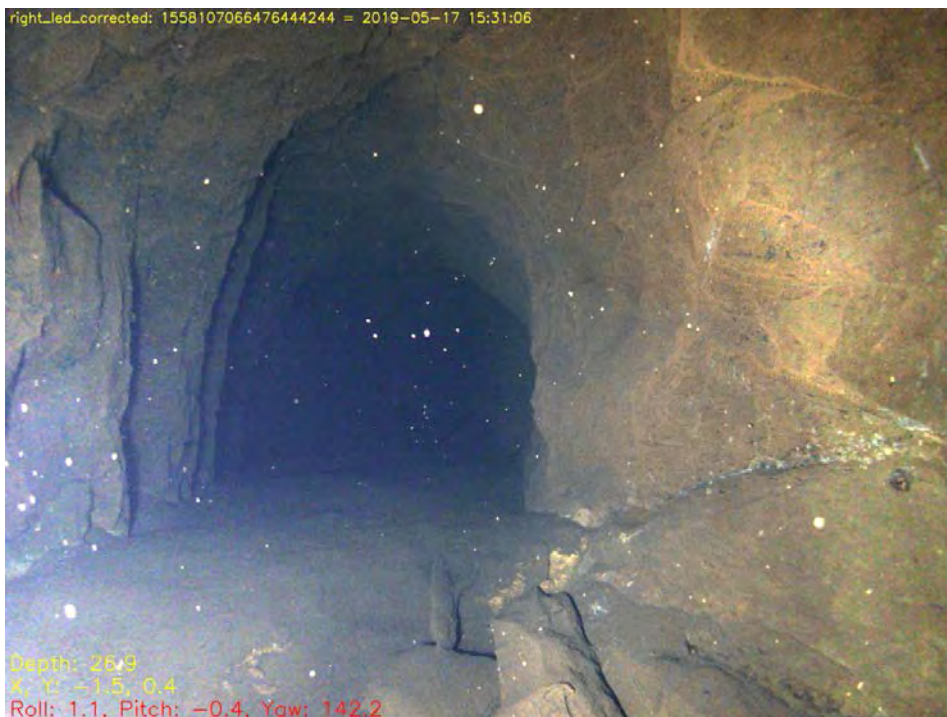
Fig. 7.24: The cross-cut to the winding shaft at PS13, has had rubble dumped on the floor after it became disused. The iron 'eye' on the wall presumably dates to when it was still in use.
