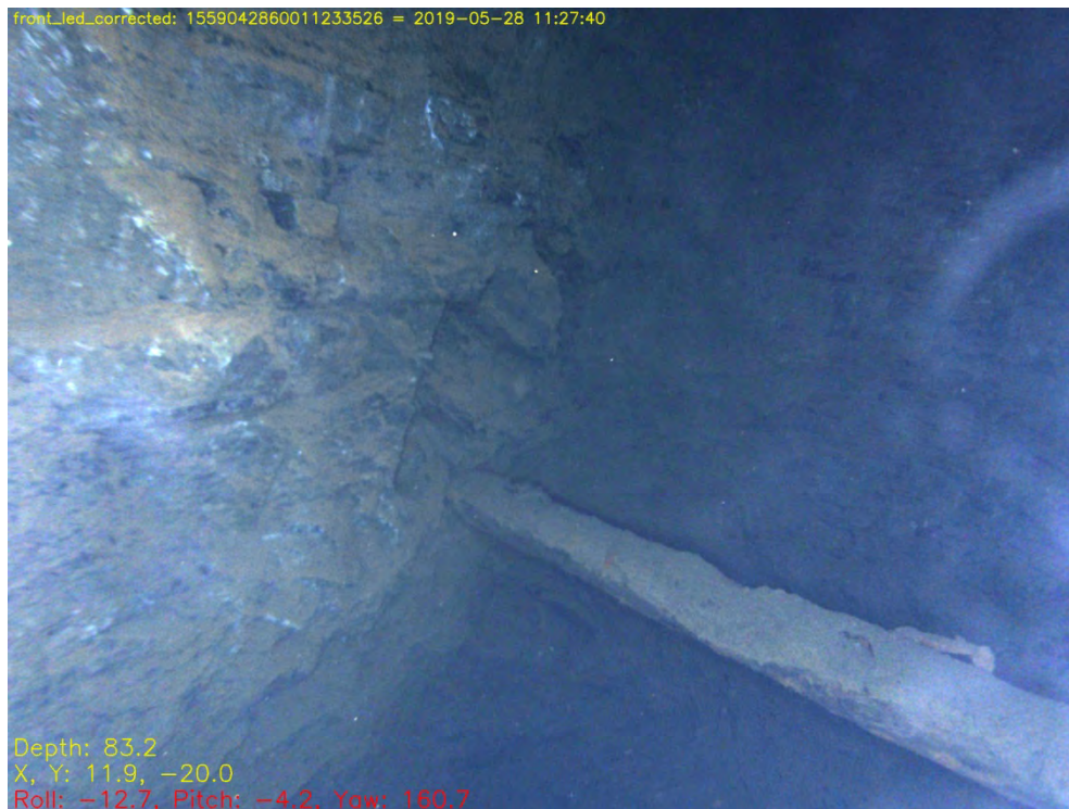
Fig. 7.66: Timbers at the north-western end of the pumping shaft were found down much of the depth explored, as here at PS14 at about -84.5m.
