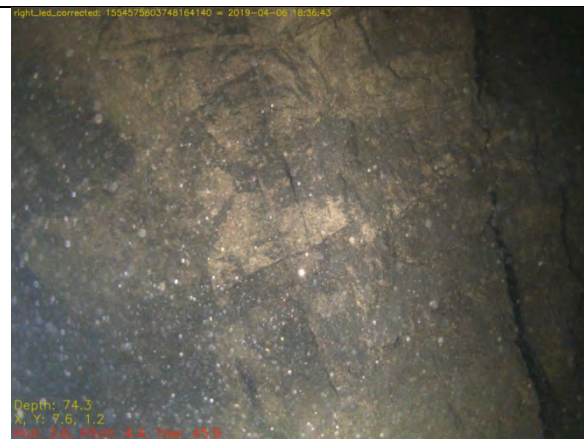
Figure 3.5 Apparent colour differentiation in granite on closer inspection is more likely to be due to varying quantities of grey sediment on differently oriented surfaces
