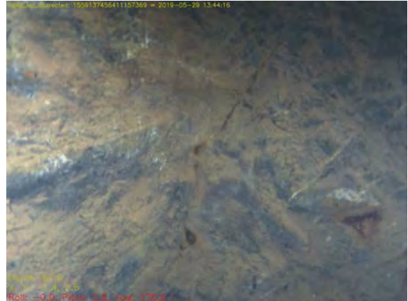
Figure 9.37: Corroding chalcopyrite mineralisation (-61.6m Winding Shaft).
