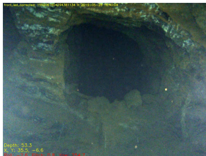
Fig. 7.56: The right-hand side passage within PW6, between c. -51.0m and c. -54.0m down. Although this superficially looks 'level-like', the 'alcove' here almost immediately enters the winding shaft, here not clearly identifiable in the gloom but seen as the submersible went forward.
