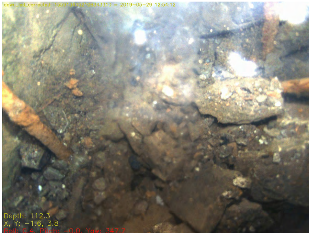
Fig. 7.68: The rubble choke (WS14) at the bottom of the accessible part of the winding shaft contains long lengths of small diameter metal pipes that have fallen down the shaft; originally they may have been part of the long set of 1788 pipes that were set on the shaft side and took water pumped up to the engine house on the ridge top for use in its boiler.
