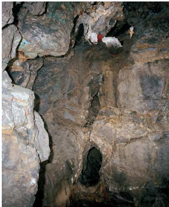
Fig. 7.49: The ‘main pipe working’ just above river level above the flooded workings, just visible at the bottom of the image, with a window into a side passage just above the water, and the ‘pipe working’ at the top of the image ascending steeply upwards from the chamber (Photograph: Paul Deakin).
