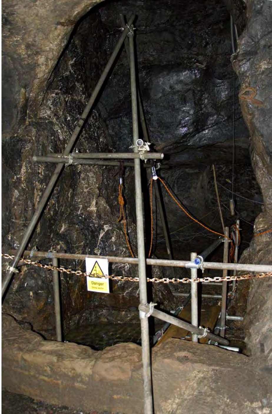
Fig. 7.36: The launch platform at the winding shaft ready for use (Photograph: John Barnatt).
