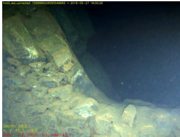
Fig. 7.58: To the right-hand side of the cross-cut to the winding shaft (PW10) at the ‘bottom’ of the lower chamber (PW6), with the adjacent protection wall (PW8) at its entrance seen here to the left, there is a large working continuing down (PW11). That this goes downwards as well as horizontally is not obvious on the sonar point-cloud data and this area need exploring more thoroughly.
