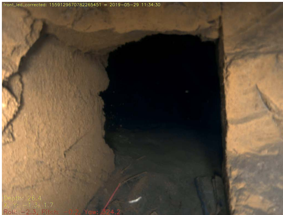
Fig. 7.41: The small level at WS2 leading off the northern end of the winding shaft, that may well lead to the pumping shaft as a cross-cut, that came here via a circuitous route and entered this at its north-western end. It can be seen to get wider, or possibly turn left, and may have been driven from the pumping shaft to bring air to the winding shaft as it was being sunk.
