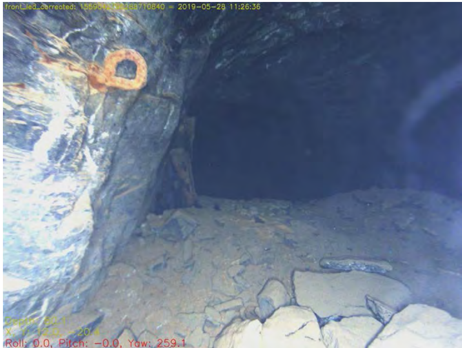
Fig. 7.24: The cross-cut to the winding shaft at PS13, has had rubble dumped on the floor after it became disused. The iron 'eye' on the wall presumably dates to when it was still in use.
