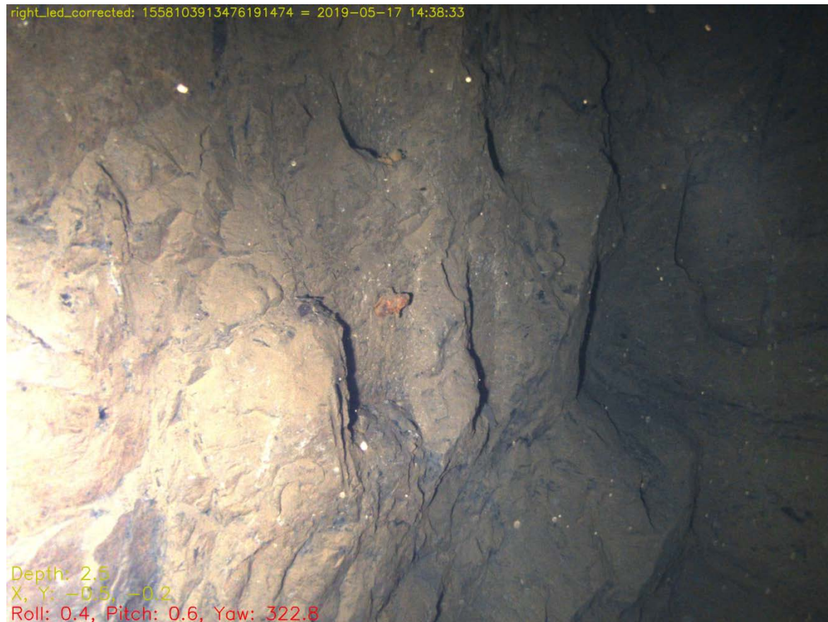
Fig. 7.34: Notches for four timbers in the pumping shaft wall at PS2, near its south-eastern end; one, at the outer edge of a platform, has had an iron pin inserted to help hold the now-lost timber in place. These timbers lay close to the shaft top and an atypically complex platform arrangement at two horizons may have existed here, unless one set of timbers was replaced by another at a slightly different depth down the shaft.
