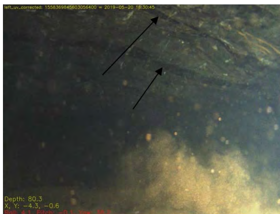
Figure 9.11: Chert beds (arrowed) in roof of cross cut between Great Shaft and Winding Shaft (-80.3m Great Shaft).
