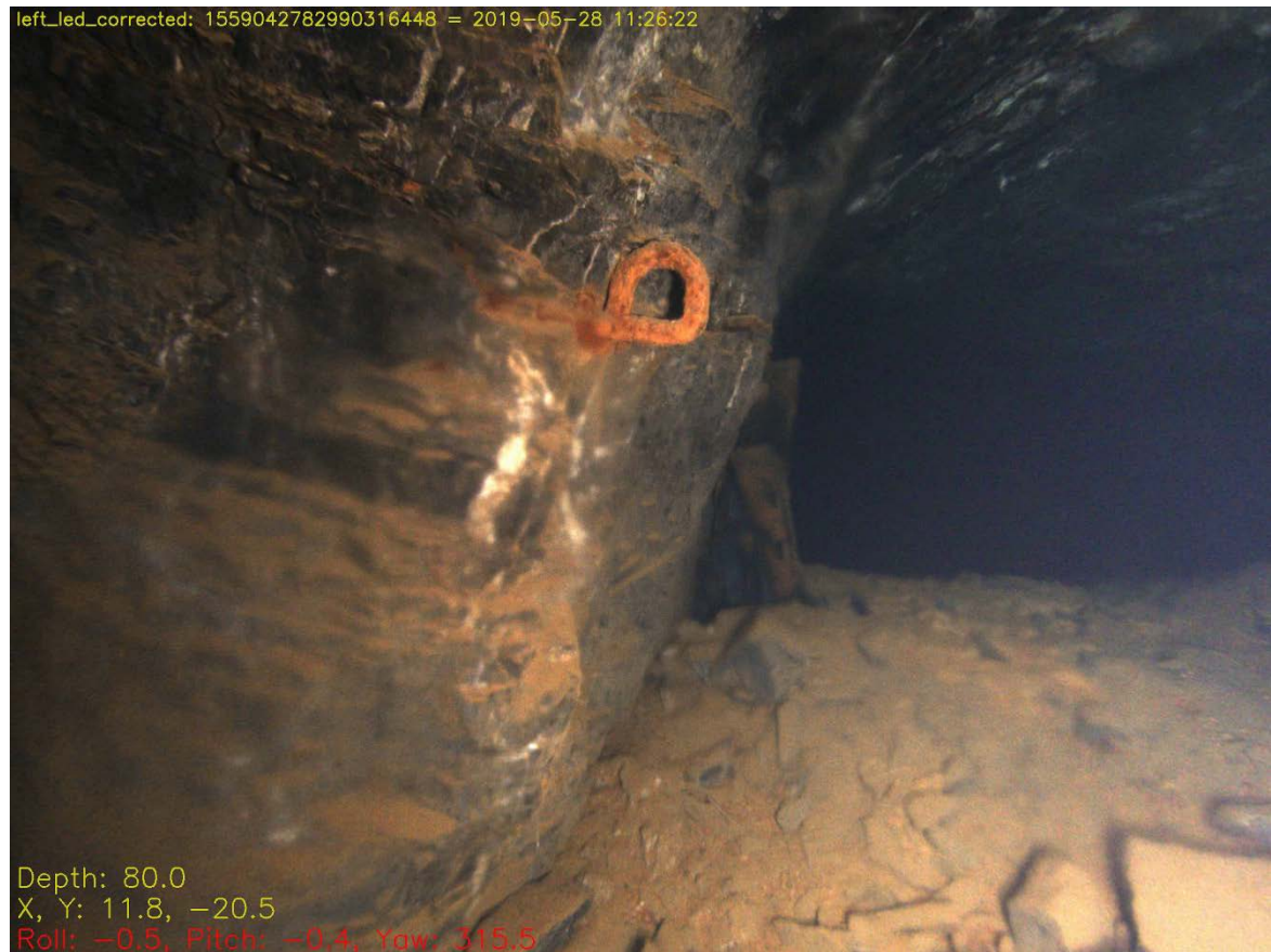
Fig. 7.35: An iron 'eye' set into the rock wall at the entrance to the cross-cut from the pumping shaft to the winding shaft at PS13. Such 'loops' are suitable for holding ropes or the tops of chain ladders, but exactly how they were used is not known.
