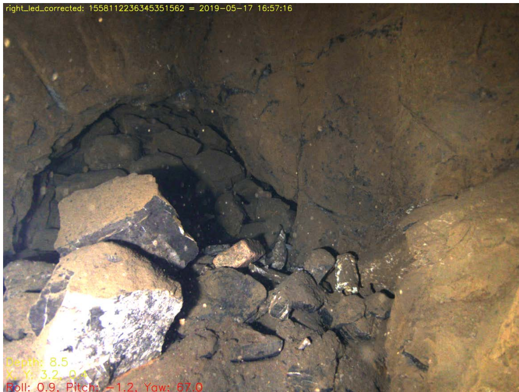
Fig. 7.26: The small level at PS3, near the top of the shaft at its north-west end, has been choked with rubble in such a way as to suggest this material came from behind the entrance, but the character of the working here is not known.
