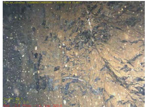
Figure 9.26: Fault or joint in anticline axis (-69.3m Great Shaft).
