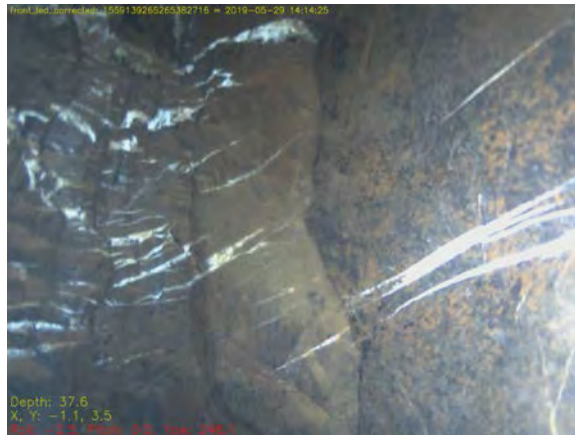
Figure 9.32: En echelon hydraulic fracturing with calcite fills (-37.6m Winding Shaft).
