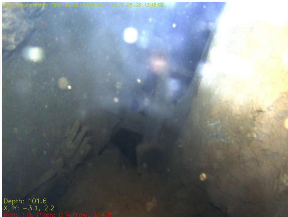
Fig. 7.39: One of the working platforms on sturdy timbers within 'side pipe working' WS11 to its left side, glimpsed only briefly through the general gloom and falling sediments; this one has waste rock above and some of its planks missing.
