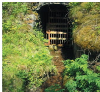
The entrance to the Ecton Deep Level tunnel.
