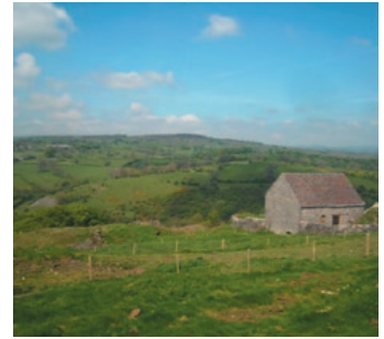
The Engine House high on Ecton Hill is a reminder of the area's rich industrial history.
